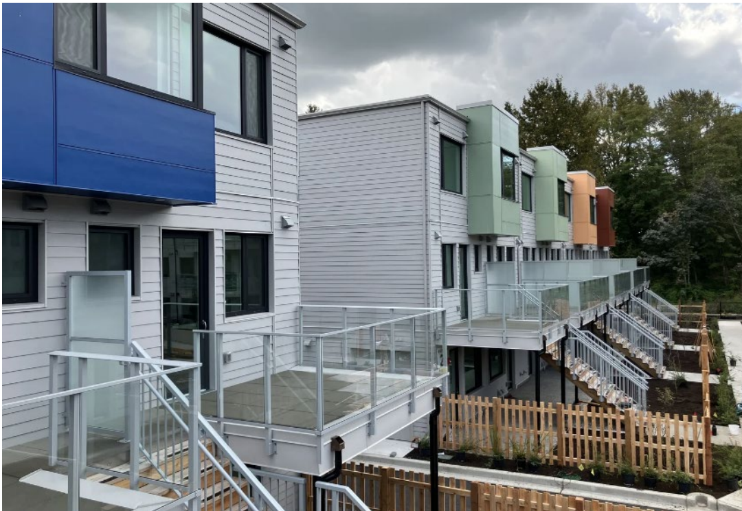
Image 10: Example of Multigenerational Housing - Xwemelch'stn, Squamish Nation, B.C.
